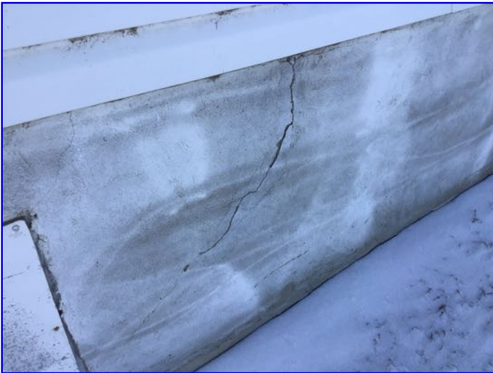
Recommend sealing cracks to prevent water entry.
