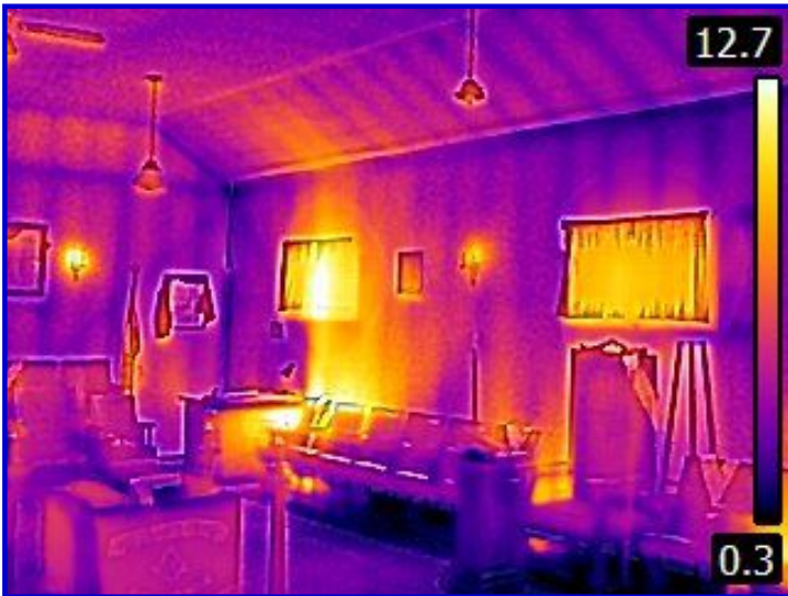
Hall Room -Thermal Image
