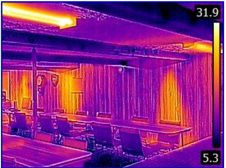
Basement right - Thermal Image
