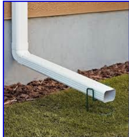
Missing downspouts observed. Suggest downspouts be installed to ensure proper drainage away from the foundation.
