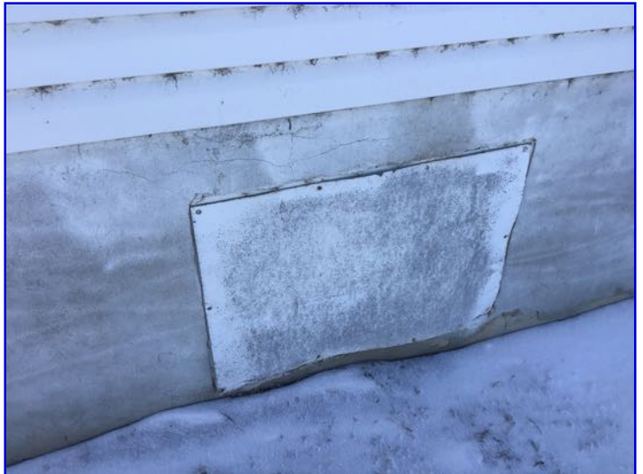
Recommend review of window patches for proper seal.
