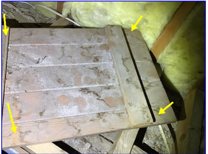
Suggest adding insulation to the back of the attic hatch, to reduce heat loss.
