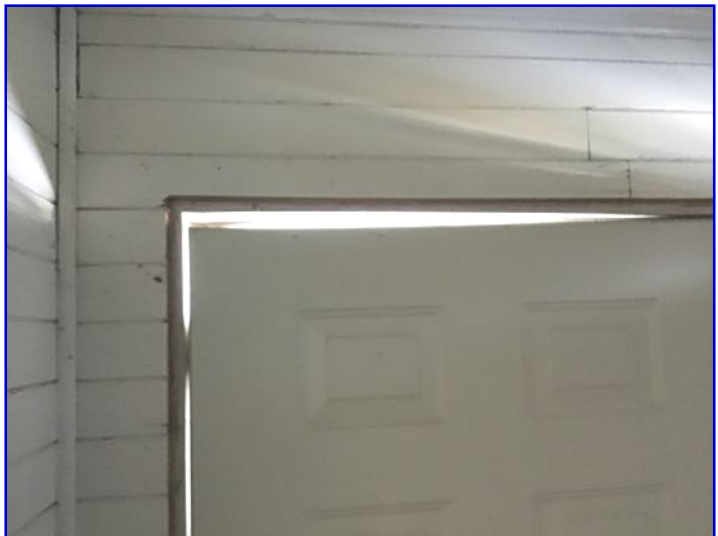
Damage / gaps noted at weatherstripping on exterior doors. Recommend replacing weatherstripping as required to prevent heat loss and pest intrusion.
