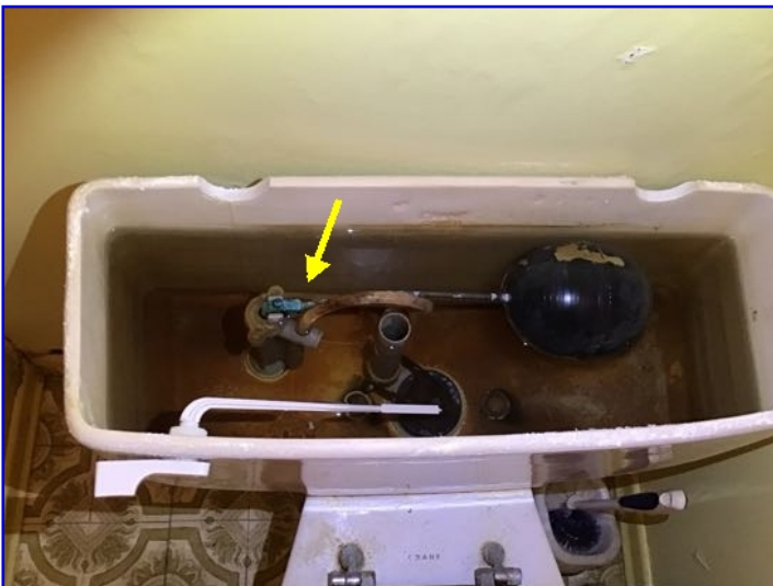
Fill valve / flapper in toilet tank causing toilet to run continuously. Requires adjustment or repair for proper flushing and to prevent water loss.
