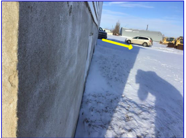
Bowing noted at foundation walls in areas.
