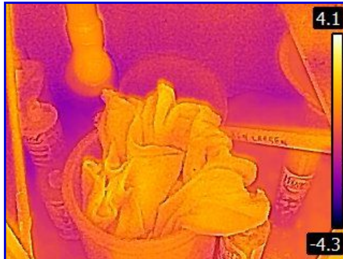
No leaking observed at Main Washroom sink cabinet on Thermal Scan
