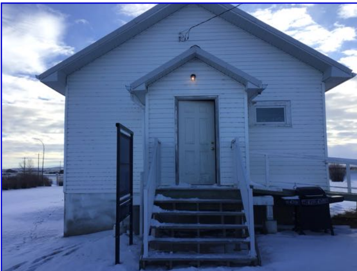
Porch is in serviceable condition.
