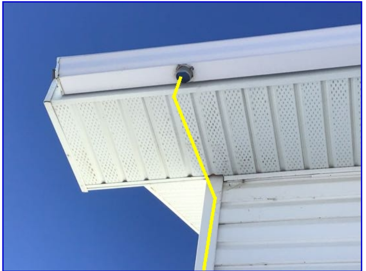
Missing downspouts observed. Suggest downspouts be installed to ensure proper drainage away from the foundation.
