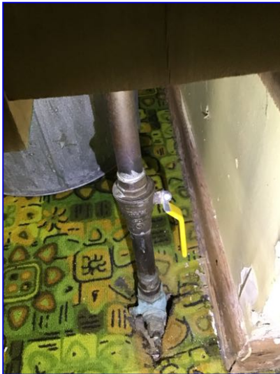
Main water shut off shown
