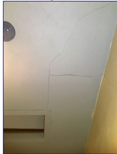
Settlement cracking noted in several walls.
