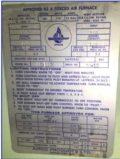
Furnace manufacturers plate
