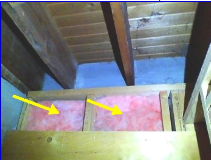
No vapour barrier noted at insulation. This can allow moisture to accumulate behind insulation batts.
