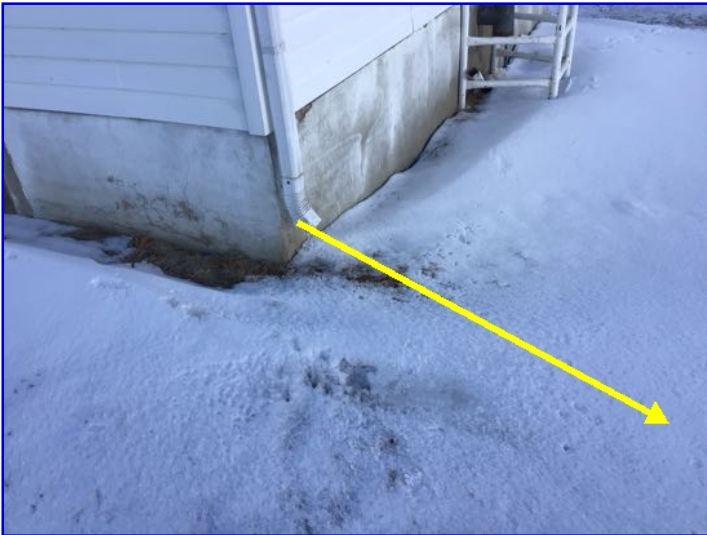
Downspout discharges water at foundation. Recommend installation of 6 foot downspout extension to ensure proper drainage away from foundation to prevent seepage.
