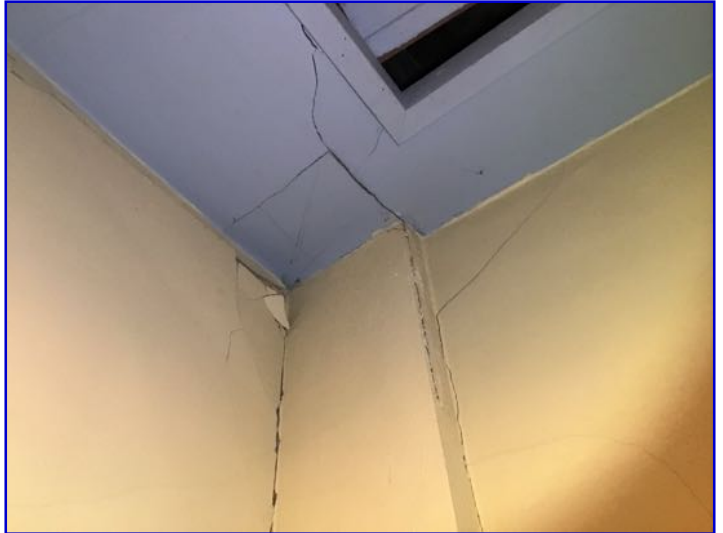
Settlement cracking noted in several walls.
