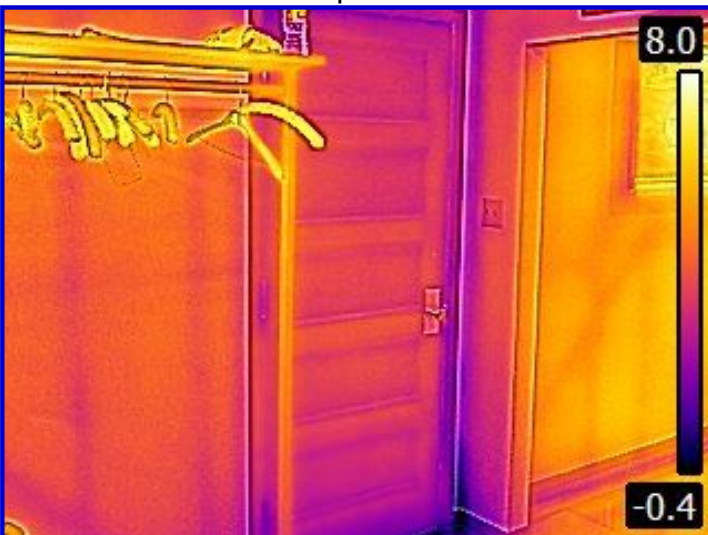
Front Entry -Thermal Image
