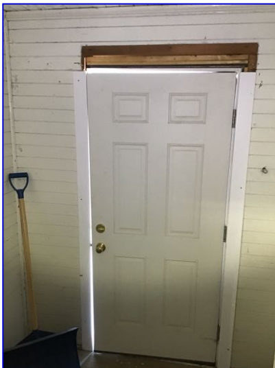
Mudroom exterior door sticks and requires force to close. Adjustments required.
