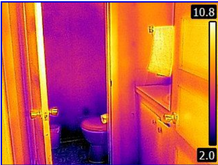
Main Washroom - Thermal Image
