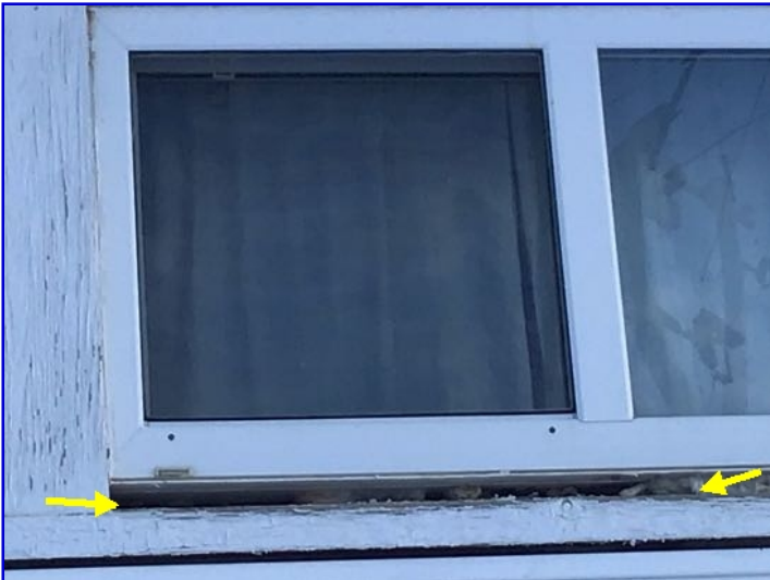
Windows poorly installed. Gaps noted. Recommend repairs
