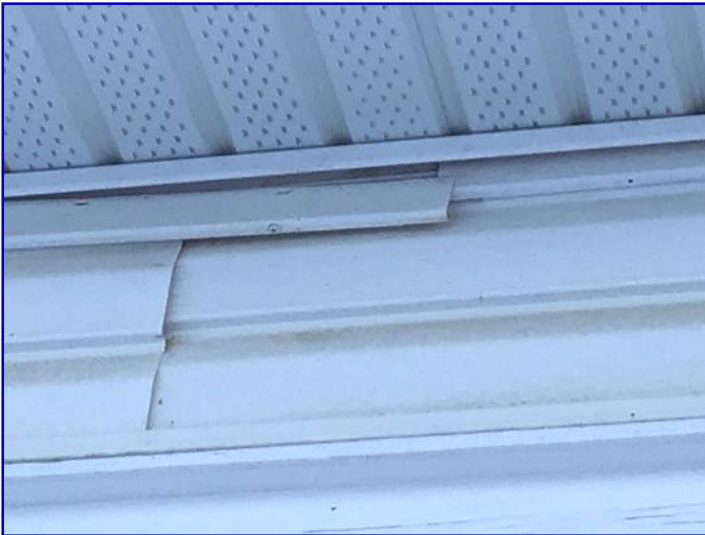
Areas os siding loose. Secure as required
