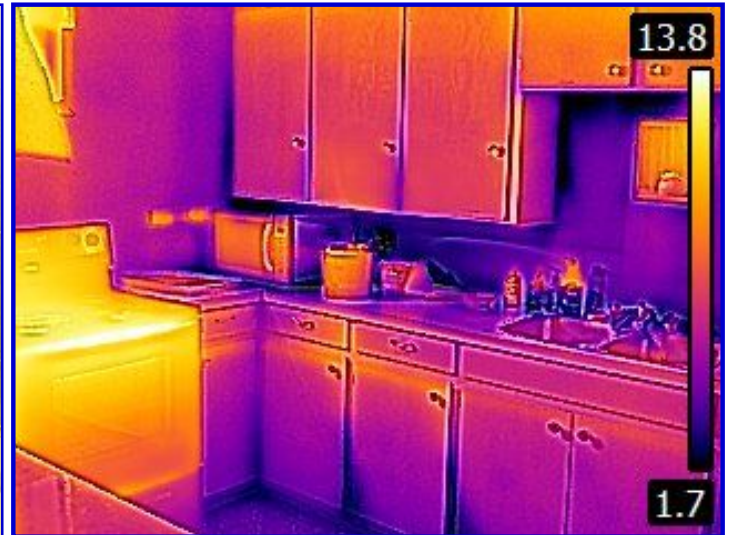
Kitchen Area - Thermal Image
