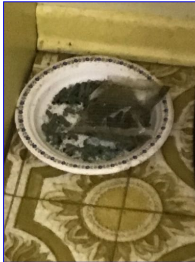
Evidence of rodents noted. Monitor for pest activity.
