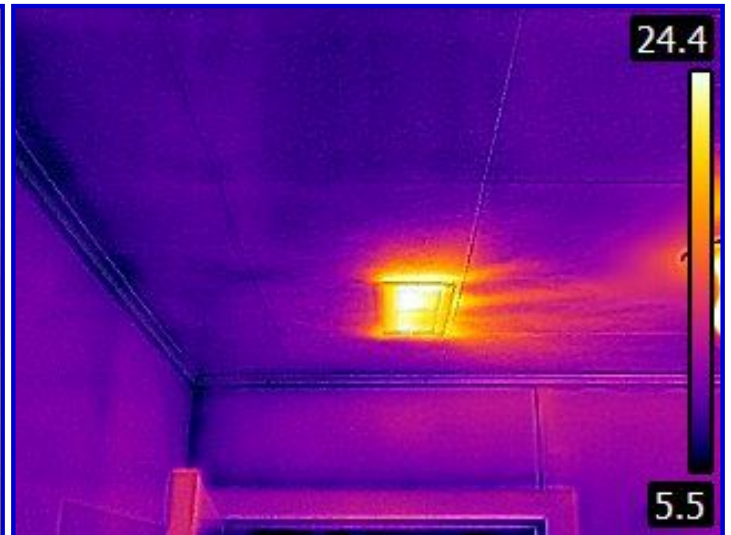
Main Washroom ceiling dry on Thermal scan
