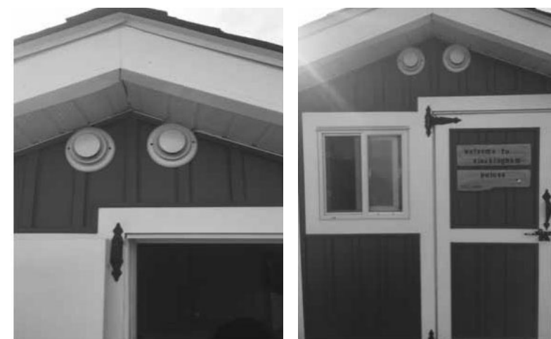
Examples of Passive Ventilation:
